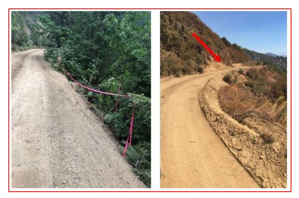
Figure 8 – Two of the soft shoulders that gave way in water tender incidents.
