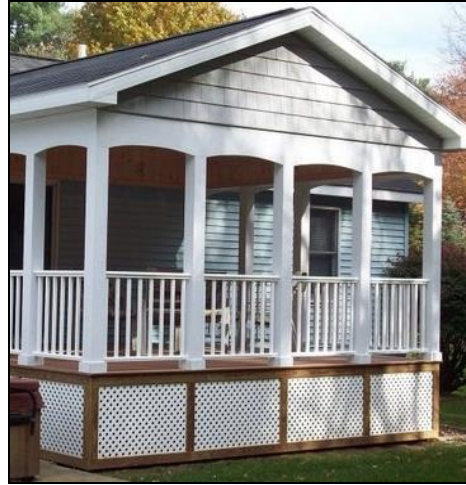
Figure 49. Screened decks restrict access from windblown debris
