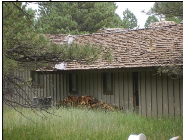
Figure 46. Significant combustible exterior fuel loads
