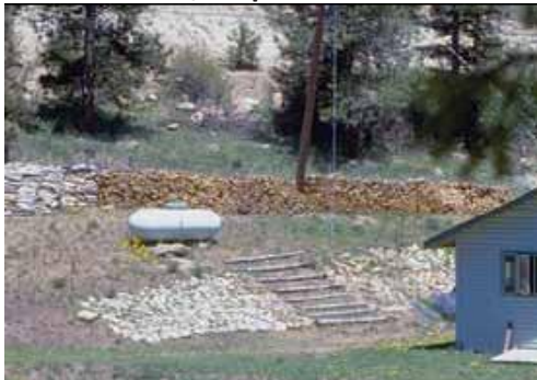
Figure 44. Example of acceptable Firewood/Propane tank location
