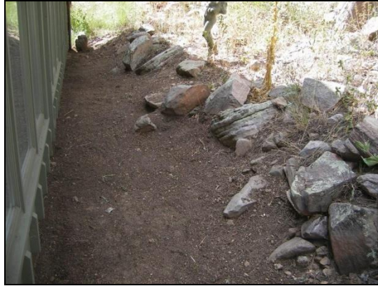
Figure 41. Effective fuel-free zone along a home's exterior
